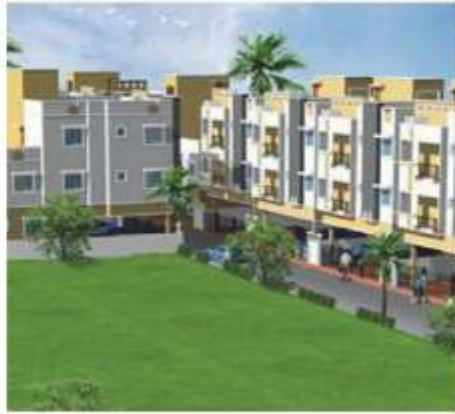
Engineered for Jeyyes Homes Perumbakkam
